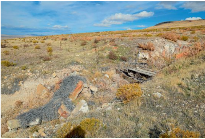
FIGURE 11. Fire, whether natural or intentional, is another threat to wooden features. This photo illustrates burned stringers on an open-deck stone culvert.
