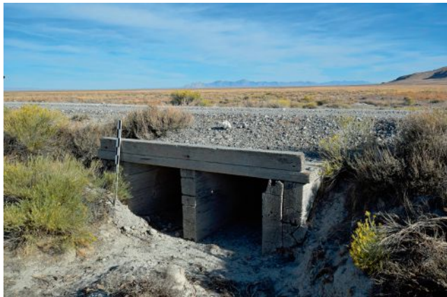
FIGURE 8. Example of a dual wooden box culvert.
