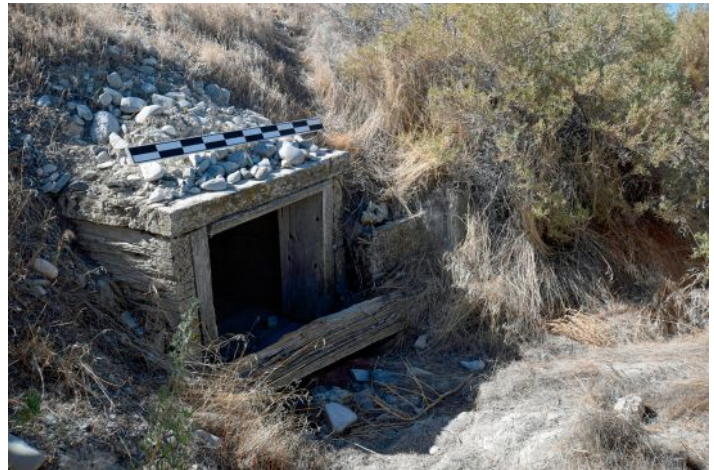
FIGURE 6. Wooden box culvert with separate horizontal strut.
