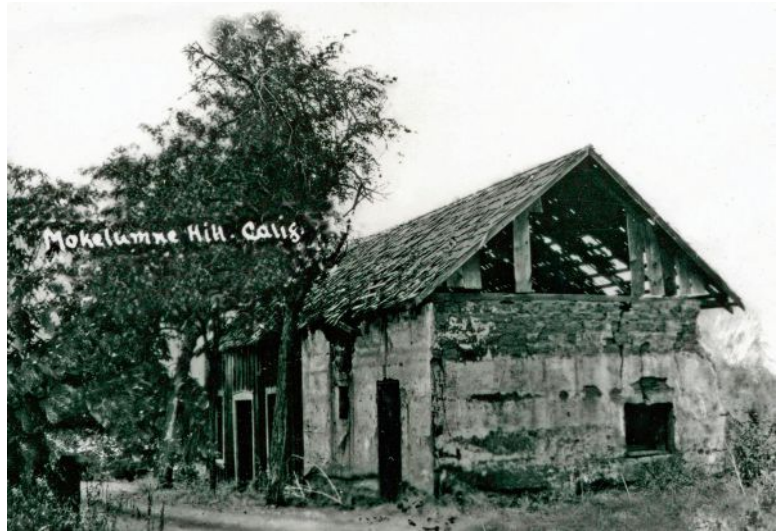
FIGURE 3. Chinatown building identified as "Adobe" on Sanborn maps (Figure 2, lot 19). (Photo courtesy of Mokelumne Hill History Society.)
