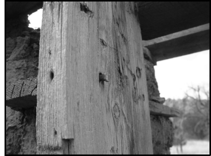
Figure 19 – Square nail anchoring door frame
