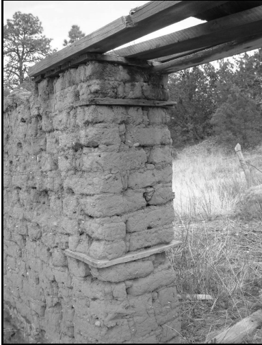
Figure 18 – Boards anchored into adobe for door frame
