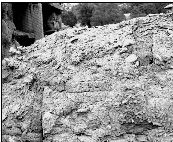
Figure 14 – Masonry – Note darker mortar
