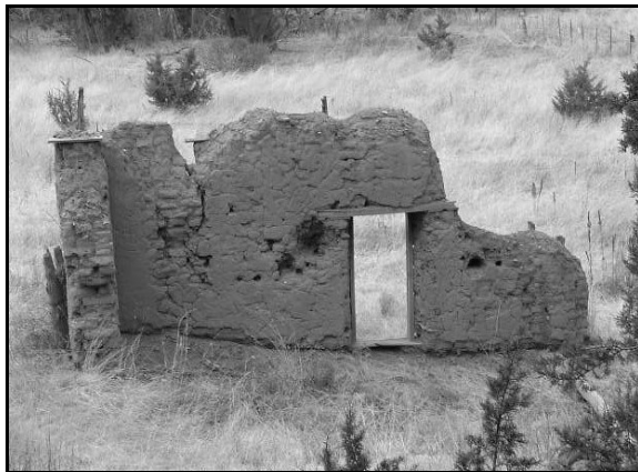
Figure 22 – West segment of front wall – back view
