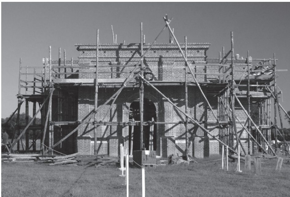
Reconstruction of the 1667 Brick Chapel with its archaeology-inspired wooden scaffold.
