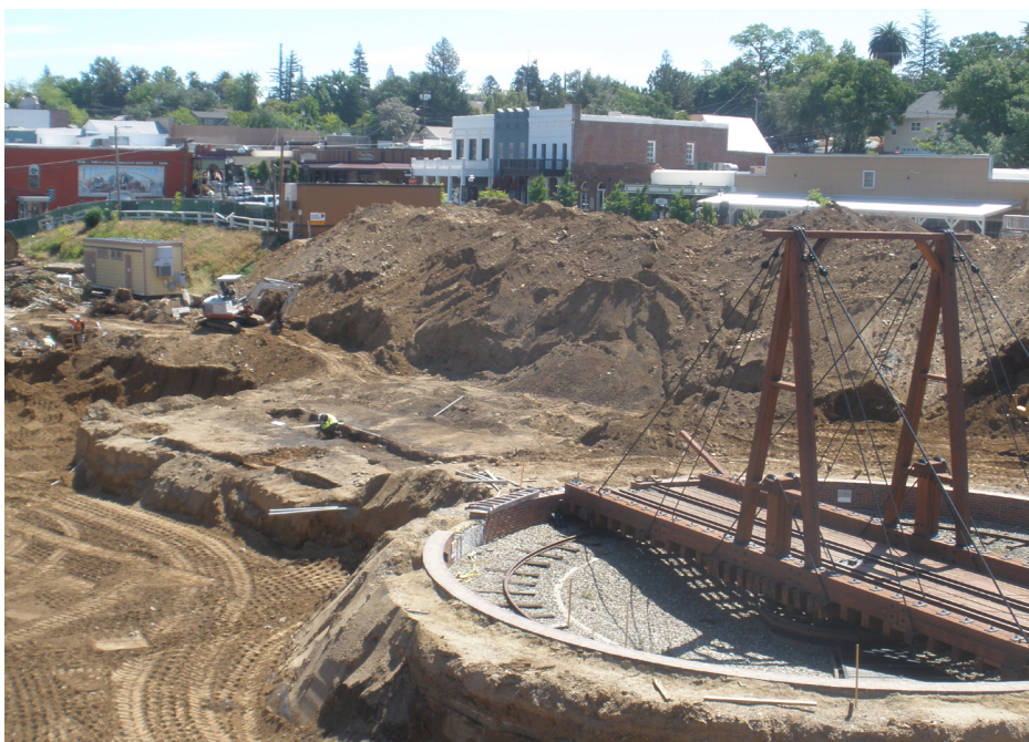
FIGURE 4. Overview of turntable (reconstructed gallows-type structure sits on historic 1854 granite pivot stone) with roundhouse excavation and inspection pit in background.
