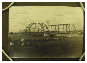
FIGURE 2. The central section of the Indian Sluice Bridge being floated into place, 1909.
