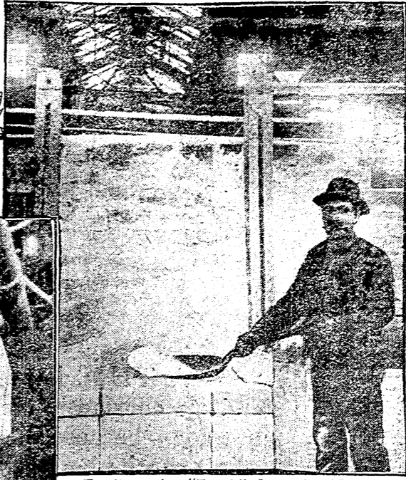
Feeding the "Batch" Into the Melting Tank, Where the Terrific Heat Registers 3,600 Degrees Fahrenheit
