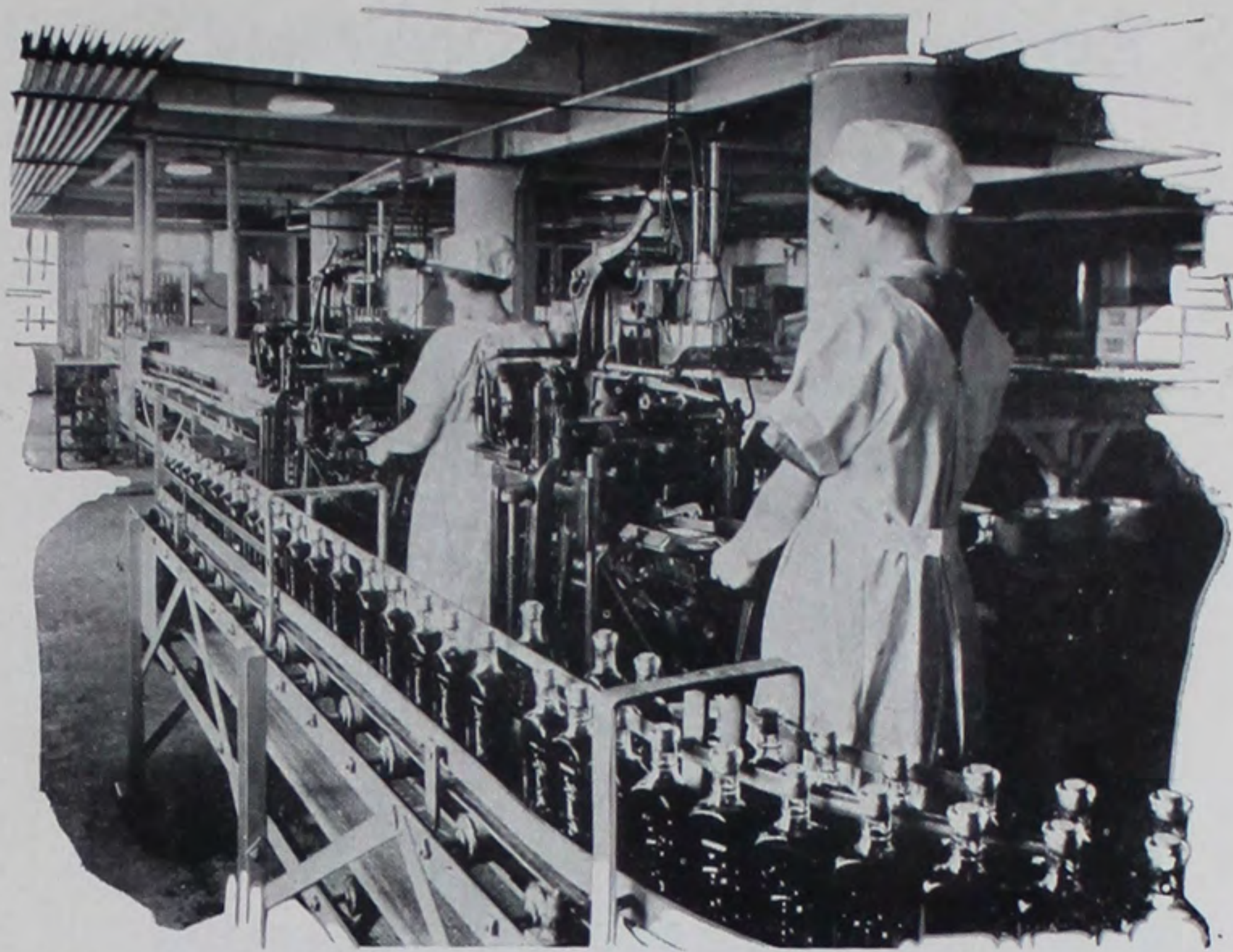
This installation solves the problem that presents itself in almost every plant where several different sizes of bottles must be labeled. Notice how the unlabeled bottles are carried to the labeling machine operators, thus insuring maximum efficiency and speed.
