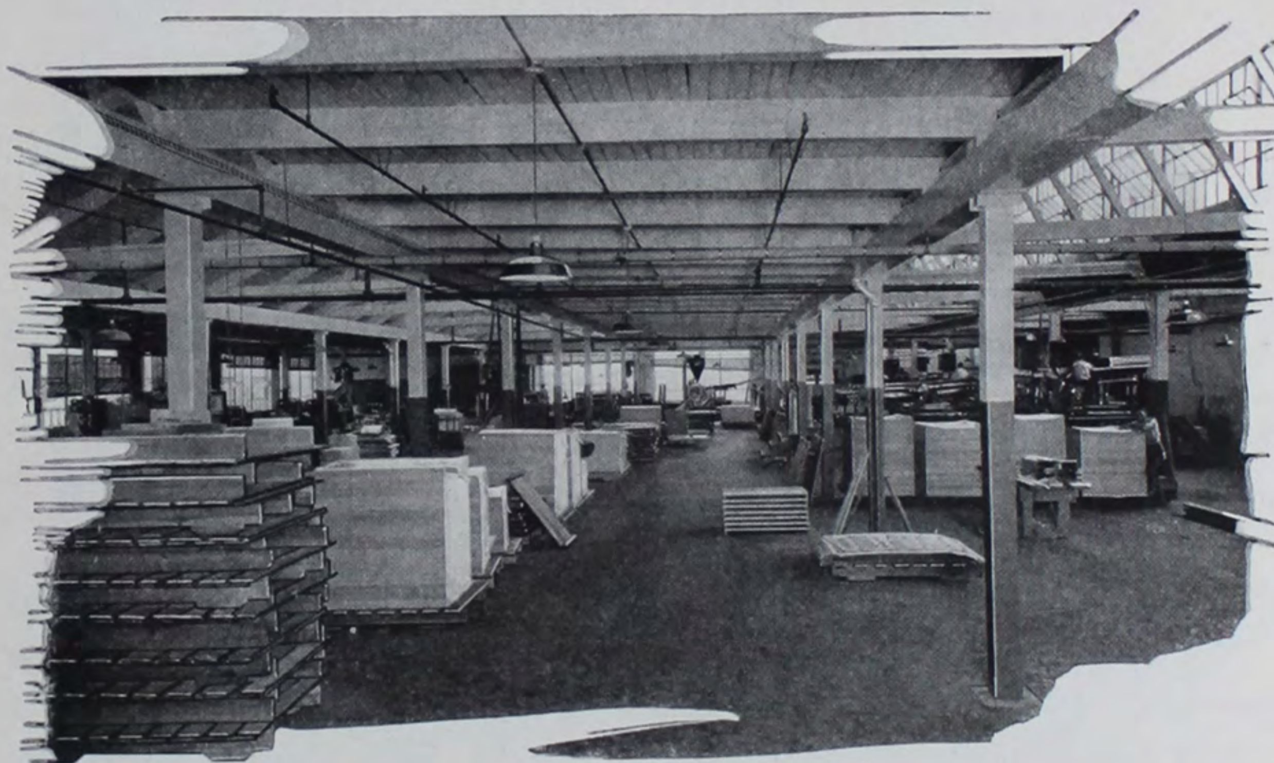
Modern construction and every device and convenience for handling stock and keeping a smooth even flow of production are found in this big plant.
